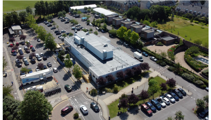
Surgical hub at Queen Mary's Hospital, St George's University Hospitals NHS Foundation Trust. Credit: Vanguard Healthcare Solutions Ltd
